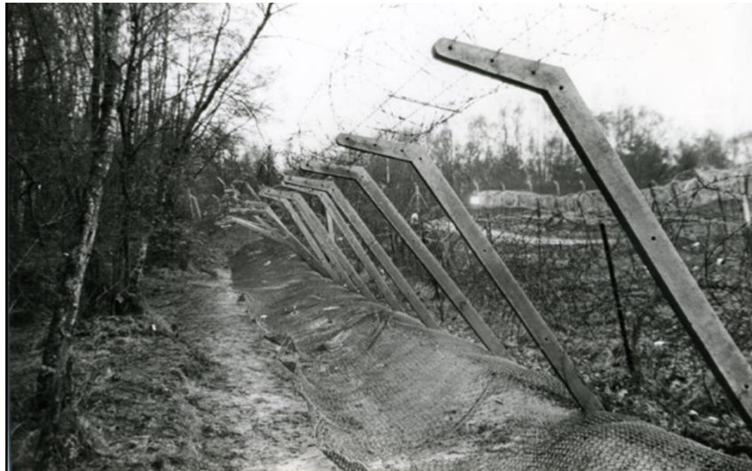
Some of the modified fence structures added to keep deer and rabbits from damaging the fence or exiting the base.
